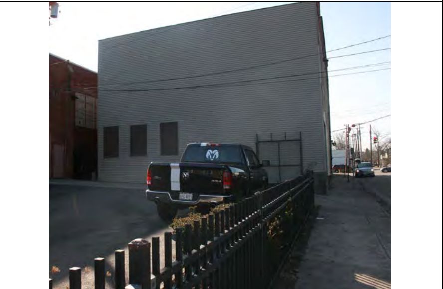
Photograph 4 – View of rear of property, looking south.
