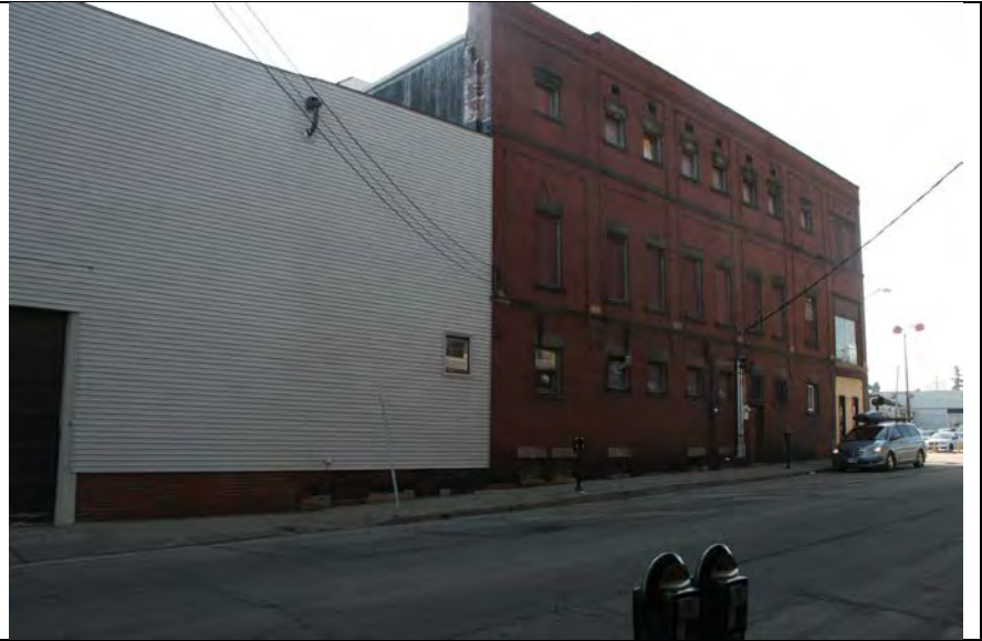
Photograph 2 – View of western elevation of Subject Property, looking southeast.
