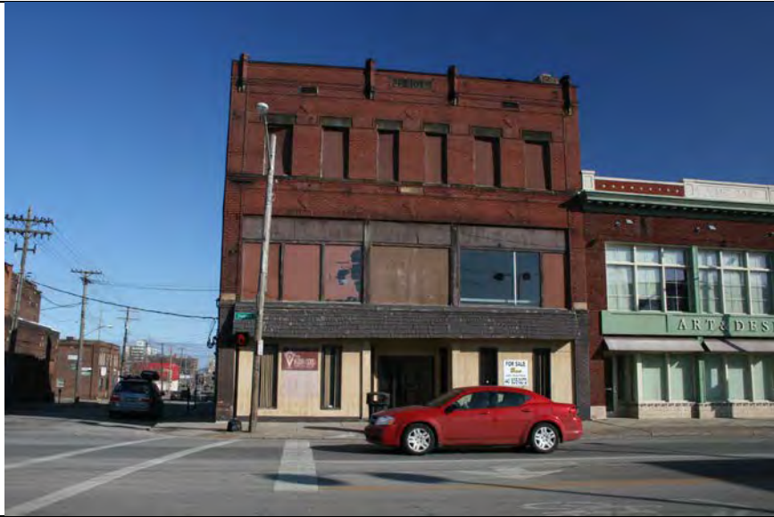
Photograph 1 – View of Subject Property looking north across Detroit Ave
