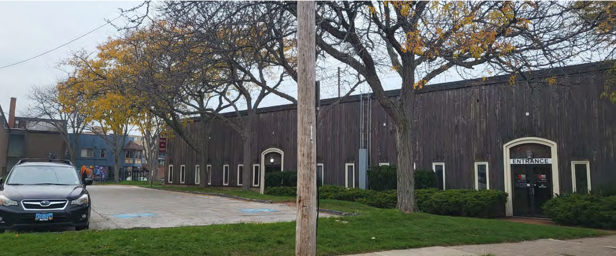
REAR OF EXISTING BUILDING
