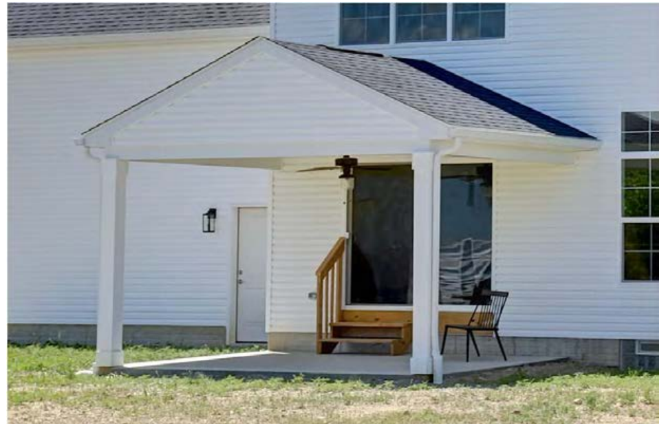
Rear porch posts (concrete slab at grade) White 1x8 PVC wrapped (Azek or similar) columns with cap and base
