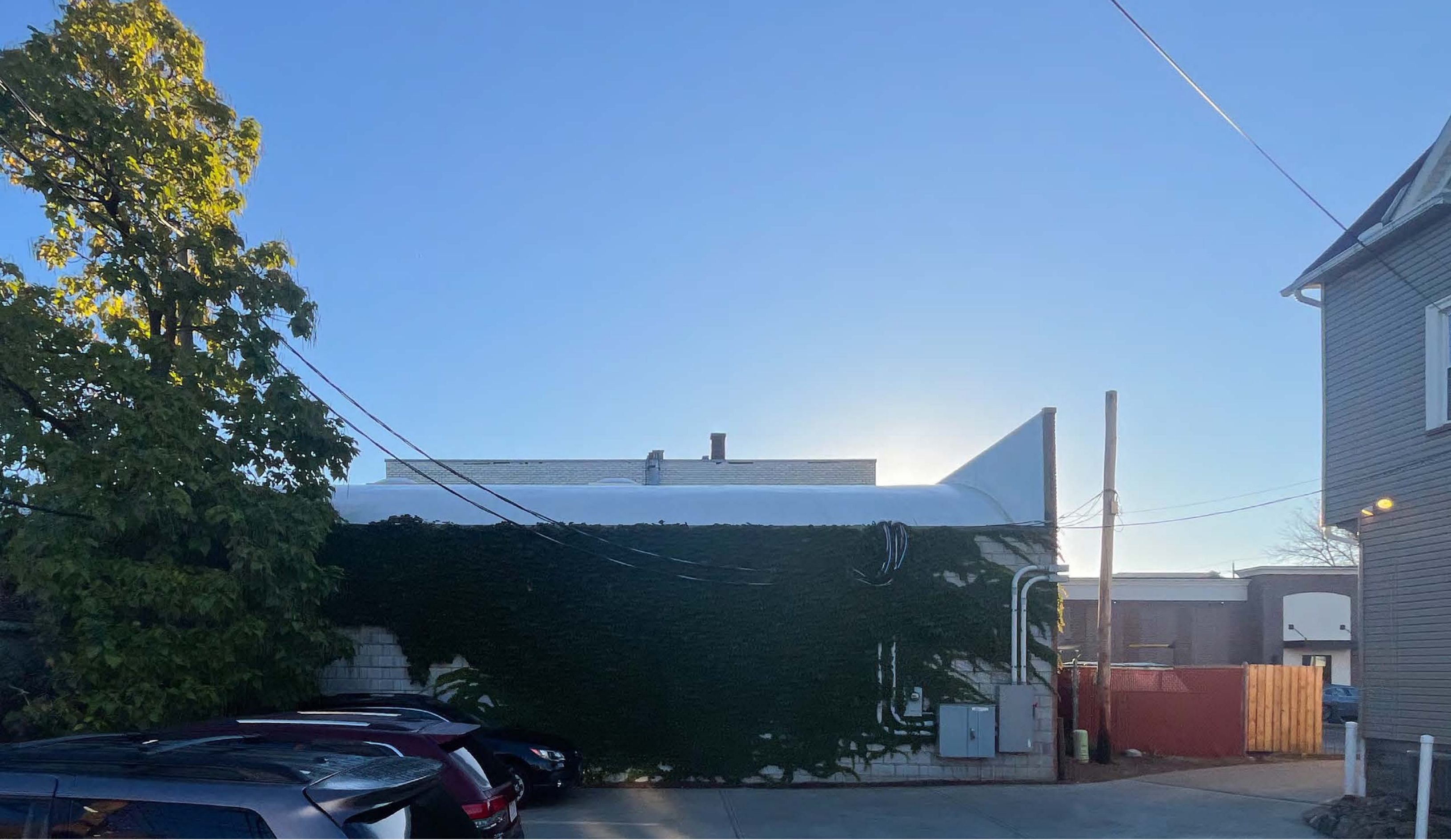
WEST ELEVATION OF ANNEX ADDITION/GYMNASIUM
