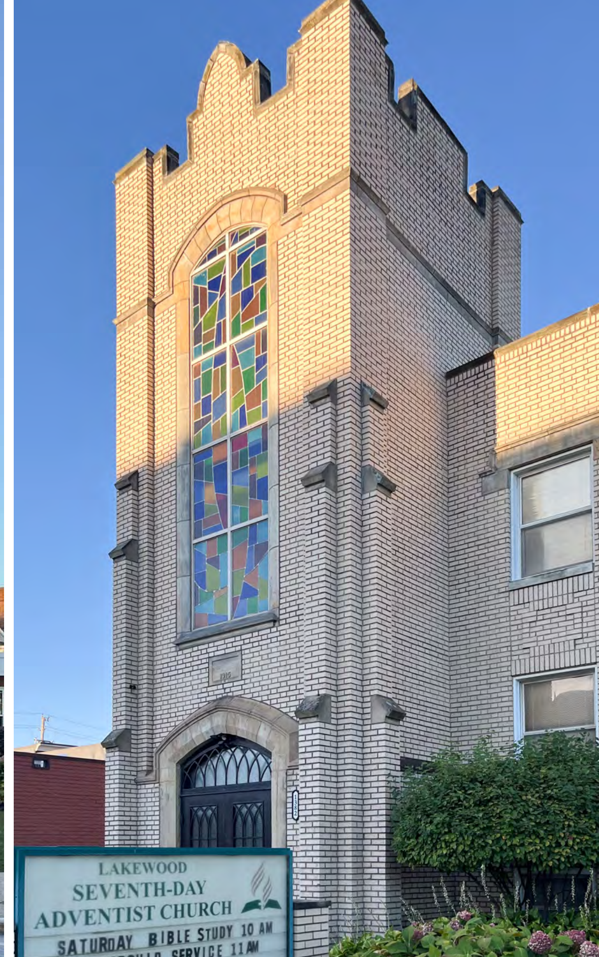
EAST ELEVATION OF SANCTUARY BUILDING
