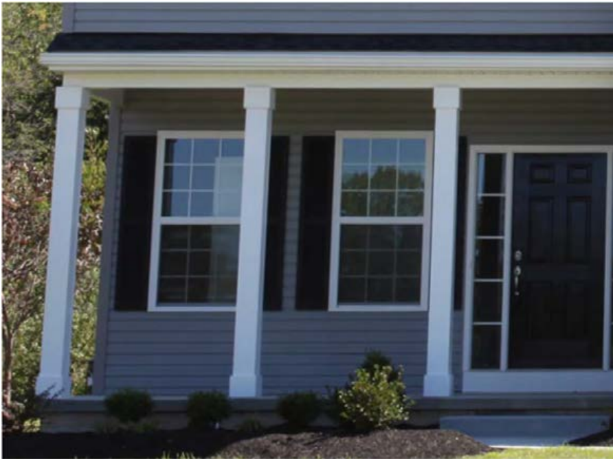
Front porch posts White 1x8 PVC wrapped (Azek or similar) columns with cap and base
