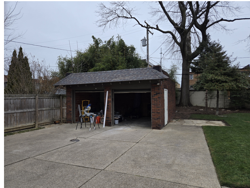
EXISTING CONDITIONS PHOTOGRAPH VIEWING NORTH N.T.S.
