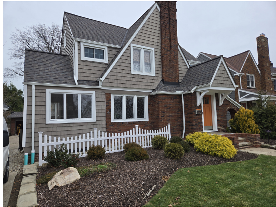
EXISTING CONDITIONS PHOTOGRAPH VIEWING NORTH N.T.S.
