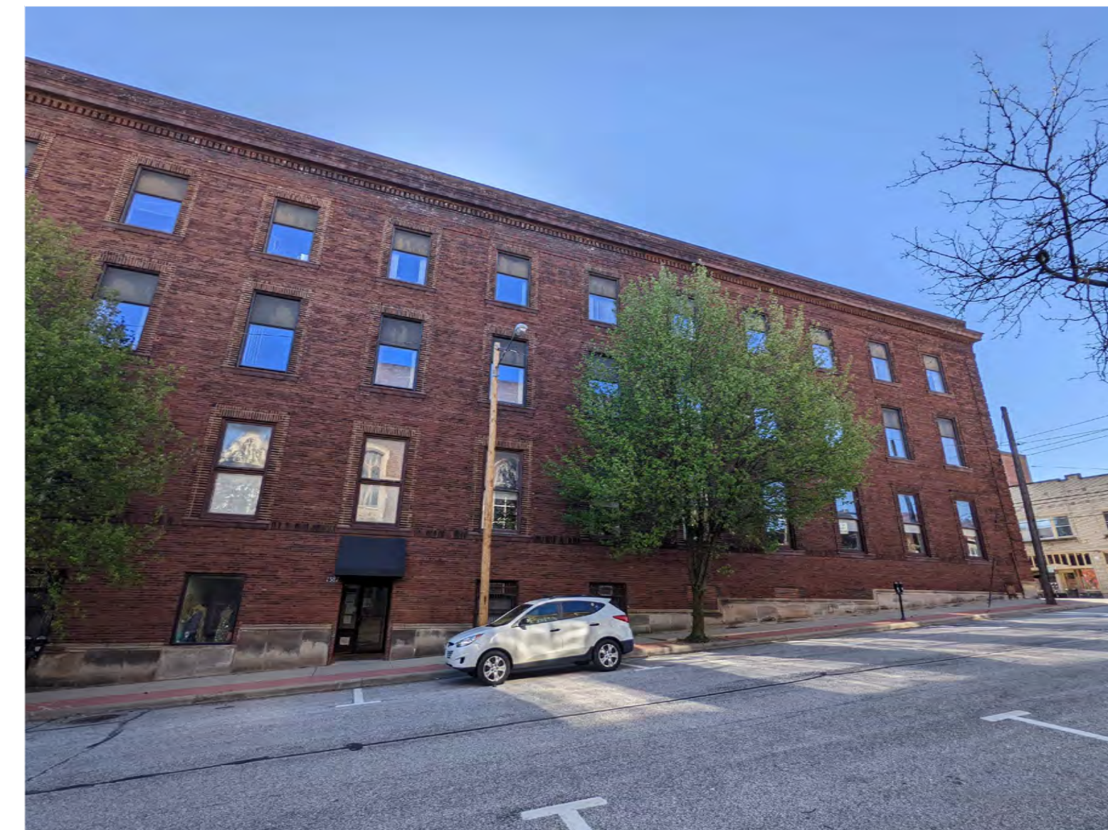
Existing Exterior Photo
