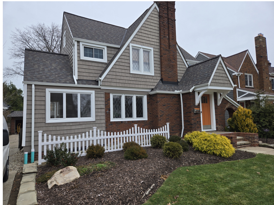
EXISTING CONDITIONS PHOTOGRAPH VIEWING NORTH N.T.S.
