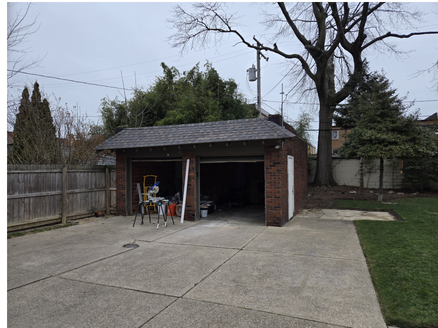
EXISTING CONDITIONS PHOTOGRAPH VIEWING NORTH N.T.S.
