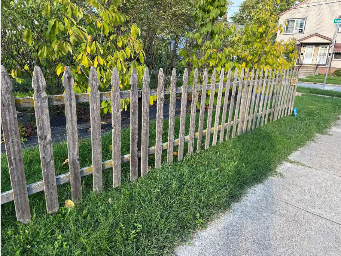
Figure 2. View of current fencing (to be removed and replaced) near intersection of Dowd and Thrush.
