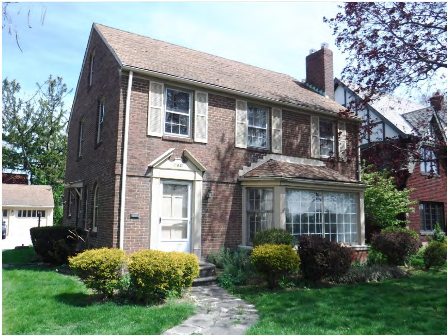
EXISTING PHOTO VIEWING NORTHEAST
