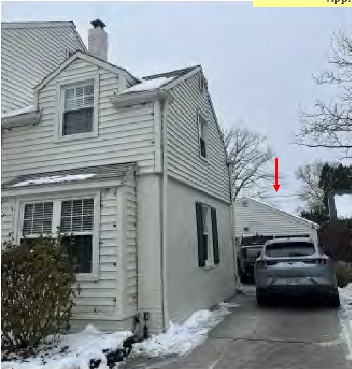
VIEW OF EXISTING GARAGE FROM DRIVEWAY
