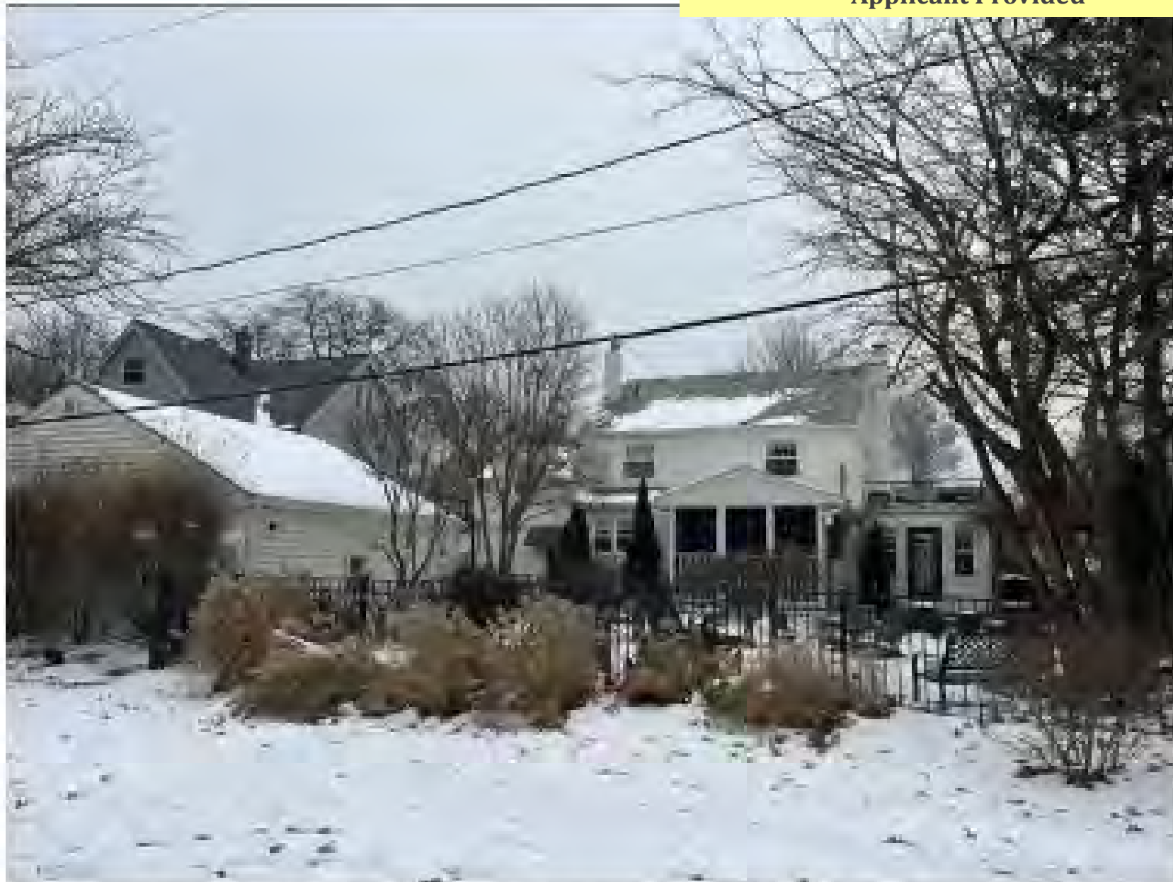
REAR VIEW OF HOUSE & GARAGE FROM PARK
