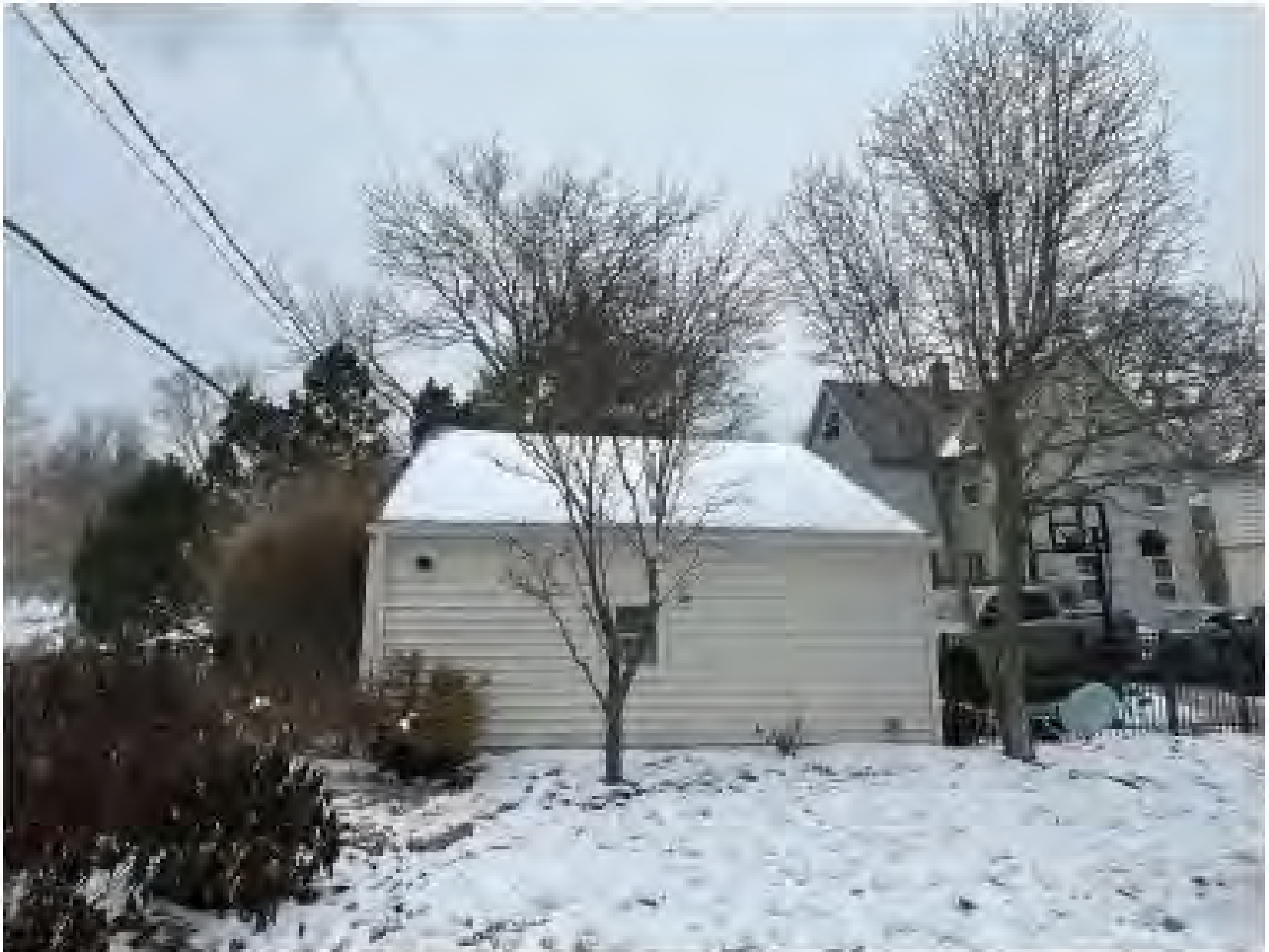
SIDE VIEW OF EXISTING GARAGE
