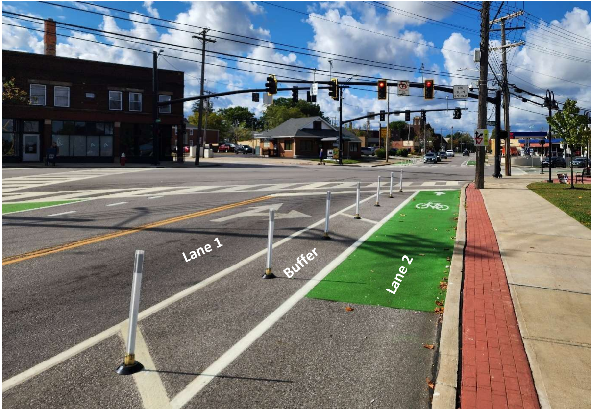
Figure 6 – Hilliard Rd Southwest Approach
