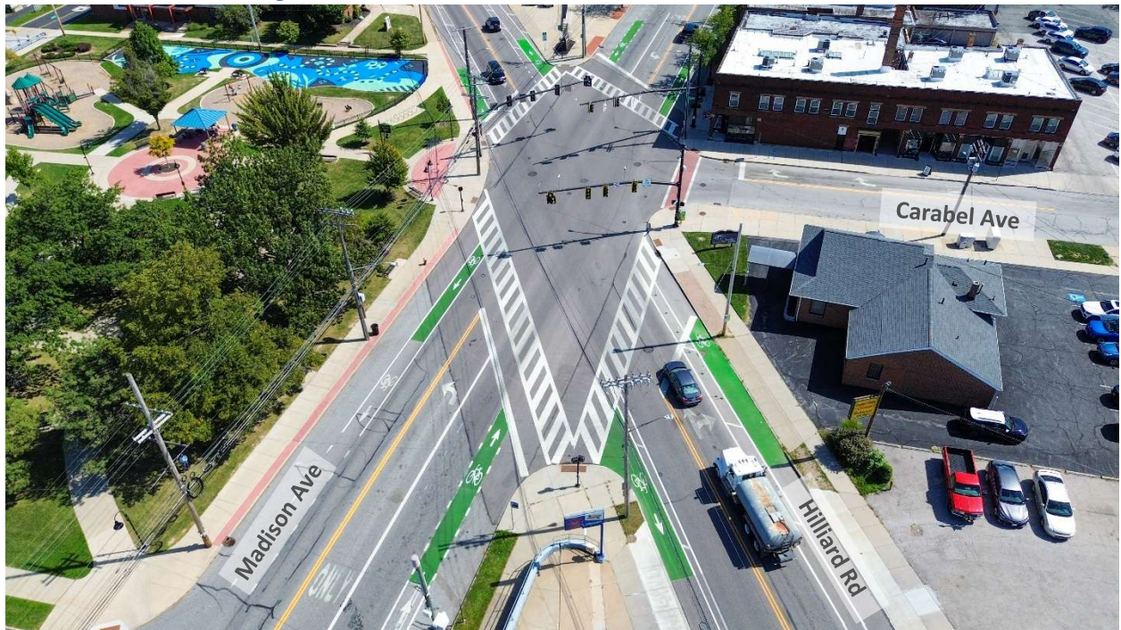
Figure 2 – Madison Ave & Hilliard Rd/Carabel Ave Aerial View
