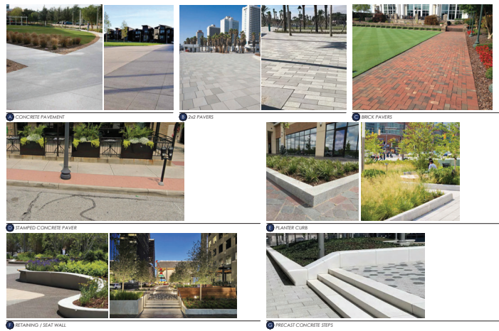
1 CONCRETE PAVEMENT 2 P&G PAVERS 3 BRICK PAVERS 4 STAMPED CONCRETE PAVEMENT 5 PLANTER CURB 6 RETAINING / SEAT WALL 7 PRECAST CONCRETE STEPS
