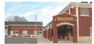
Harrison Elementary Source: City of Lakewood
