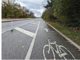
Figure 16. Protected bikeway on Clifton Boulevard
