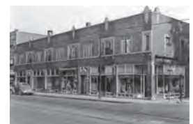
Figure 13. View of Detroit Ave in 1934 (Source: Cleveland.com)
