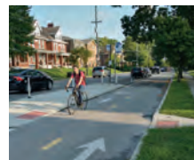
Figure 39. Floating bus stop along parking protected bike lane (Toole Design)
